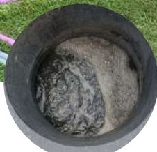
Reactor 2 MBBR. Reactor for Nitrification.
